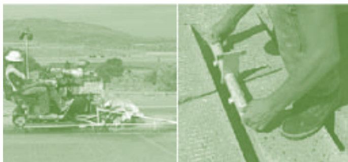
(right) inserting dowel
